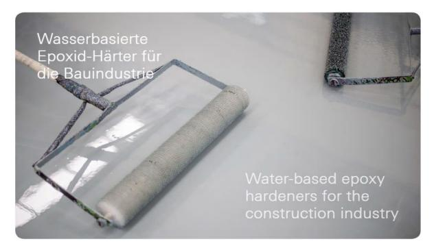
Water-based products have also come to play an ever increasing role in construction chemistry. VARENA CHEMICAL has succeeded in developing a water-based epoxy resin hardener that is suitable for use in primers, EP mortars and EP floor coating systems.
